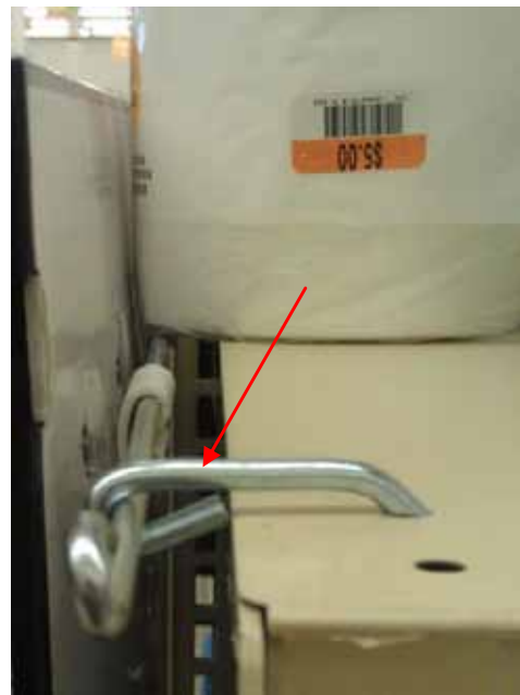
Power bar support hung on shelf structure.
